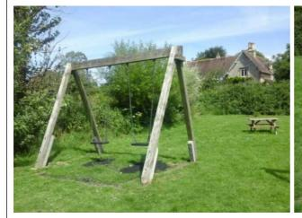
The timber has a number of air cracks apparent, the splits will have penetrated the preservative applied to the timber and allow Finding: water ingress to the unprotected areas
