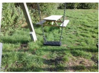
**Finding:** The picnic table forms a hard object within the falling **Action:** Re - locate the picnic table space of the equipment in contravention of the requirements of BS EN 1176 Part 1
