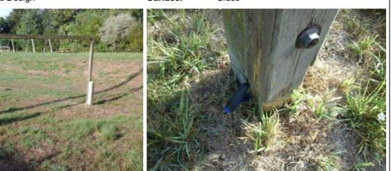
**Finding:** There are areas or parts of the timber on the structure that have rotted
