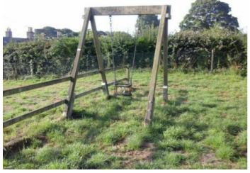
Finding: The posts on the swing barrier are slightly loose in the ground
