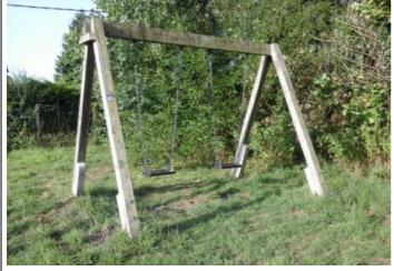
Finding: The seats are too close to the frame as defined in BS EN 1176 Part 2; this is a low risk failure and no remedial action is required
