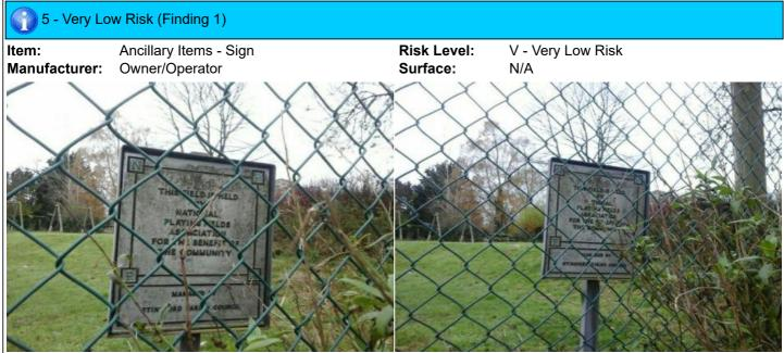
**Finding:** BS EN 1176 Part 7 recommends that signage shall **Action:** Provide additional information include emergency contact details and contact details of owner / operator for reporting maintenance issues
