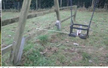
**Finding:** BS EN 1176 Part 2: Annex A makes a recommendation that fences or enclosures should be up to 1.50m from the edges of the swing seat to the sides, and subject to risk assessment, from the edge of the impact area. This is however, a low risk finding and no remedial action is recommended.
