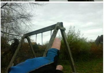
**Finding:** A number of fixing(s) have worked loose, the cross **Action:** Secure all loose fixings bar moves when in use
